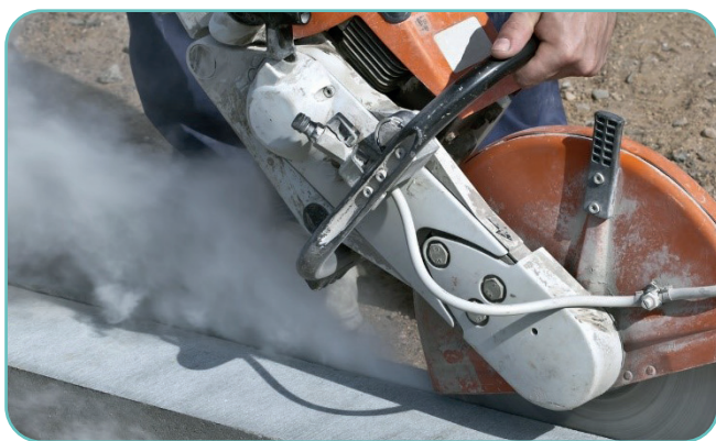
Figure 1-6: Cutting concrete block Source: BNP Products
