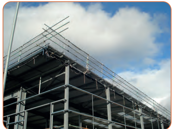
Figure 7-74: Safety nets under partially completed roof. Source: RMS.
