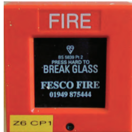
Figure 4-37: Fire alarm call point. Source: RMS.
