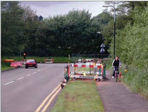
Figure RSP-3: Risks from roadside work.
