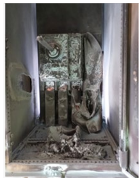
Figure 10-2: Electric arc damage in 415v switch panel - tools melted at front, hole where the left-hand panel vapourised
