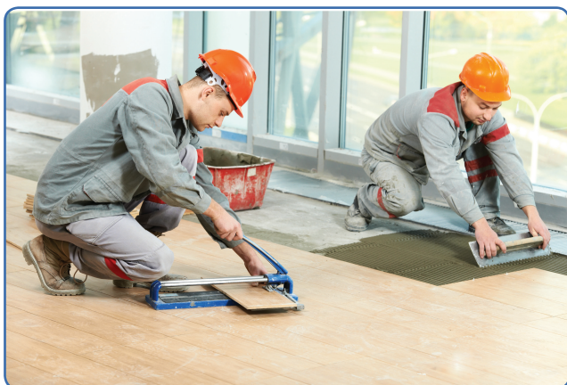
Figure 1-3-2: Contractors working at occupied premises. Source: Shutterstock.
