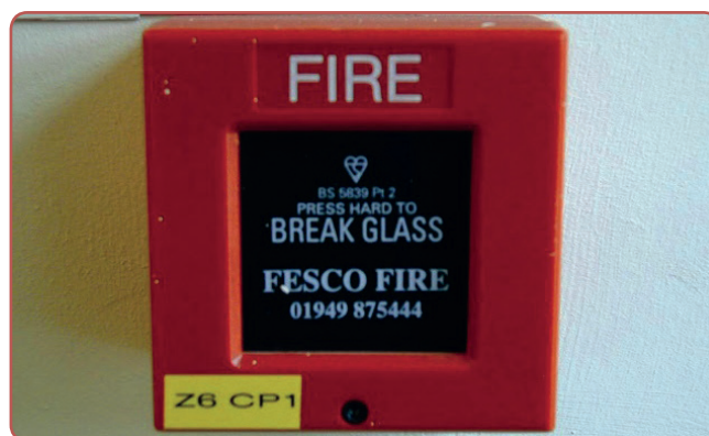
Figure 2-6-48: Easy operation alarm call-point. Source: RMS.
