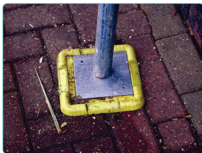
Figure 2-1-45: Base plate and protection. Source: RMS.
