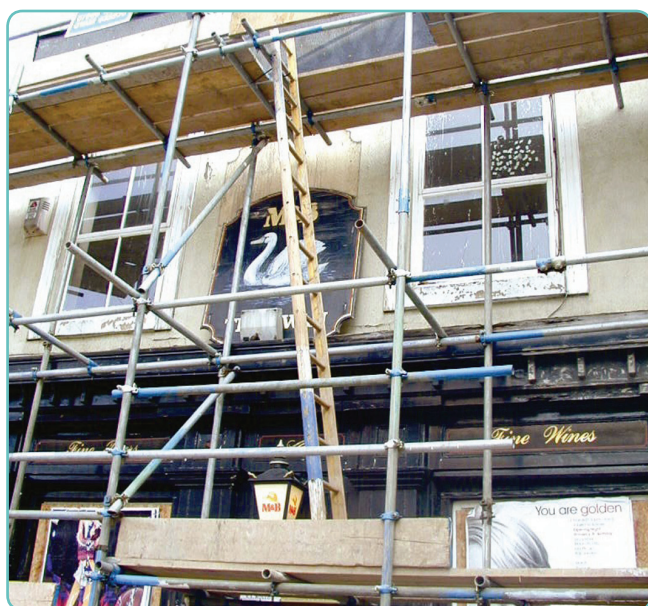
Figure 2-1-43: Independent tied scaffold. Source: RMS.
