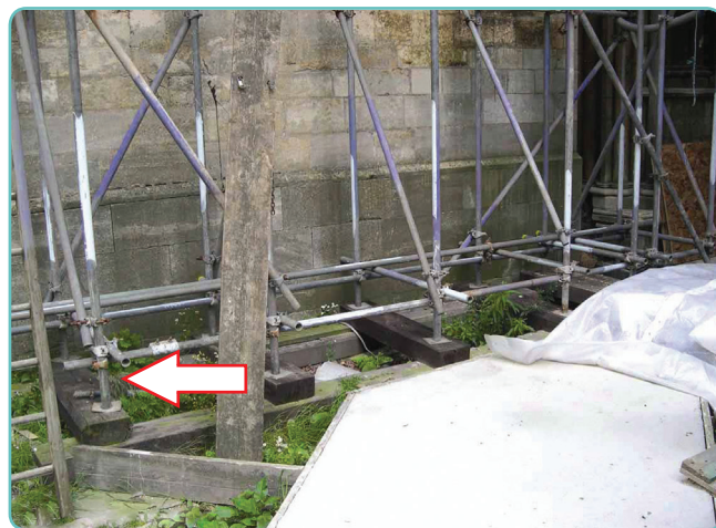
Figure 2-1-44: Base plates and sole boards. Source: Lincsafe.
