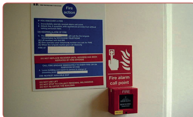
Figure 2-6-49: Alarm point identified and well located. Source: RMS.
